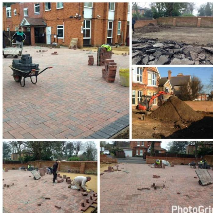
We have now completed the project to improve the area in front of the main Approved Premises building. This has involved the removal of a number of trees, a new front wall opening up a second entrance/exit and a new car park surface being laid. The result is a larger parking area with defined spaces and a more attractive aspect.
